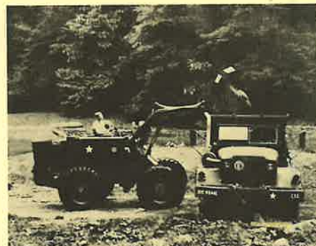
Swimming pool fix-up at Horse Creek Recreation Center.
